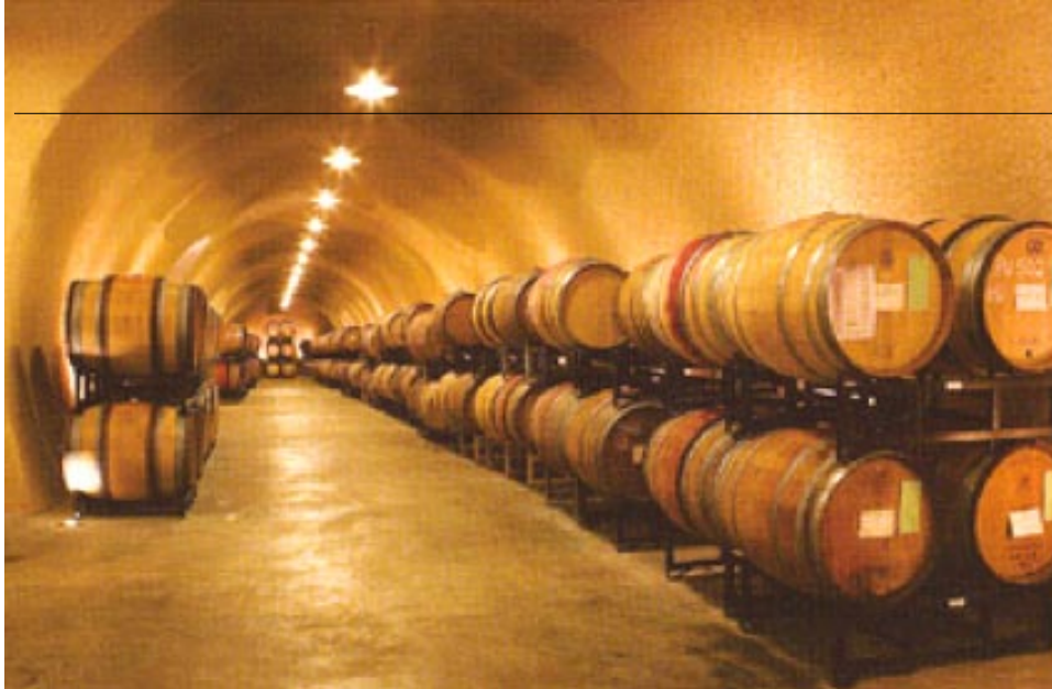
The Lynmar Winery cave consists of seven bores (the longer shown above) that feature integral color shotcrete, ambient overhead and dramatic back lighting of the barrels, and a sloping "W" concrete floor with stainless steel floor drains.
